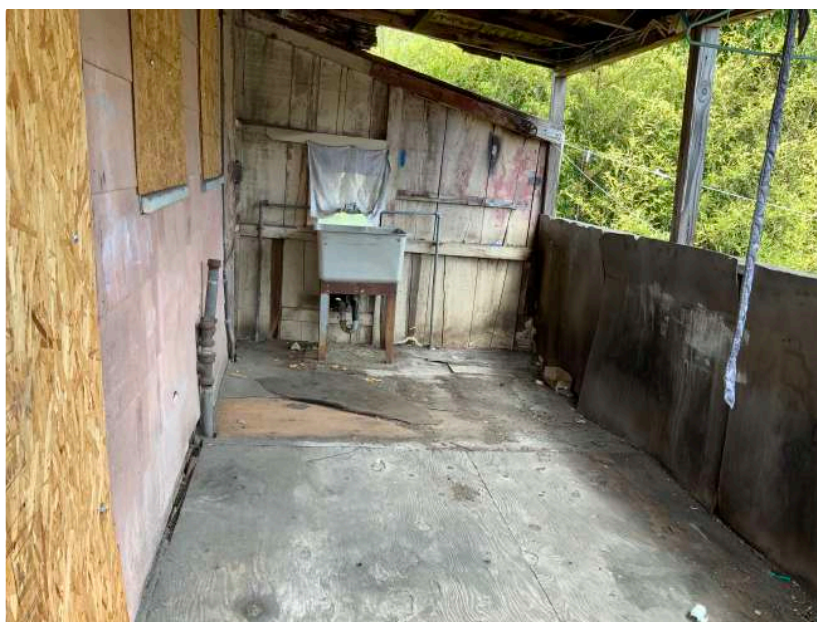
Subject Property; Exterior Deck; Facing North
