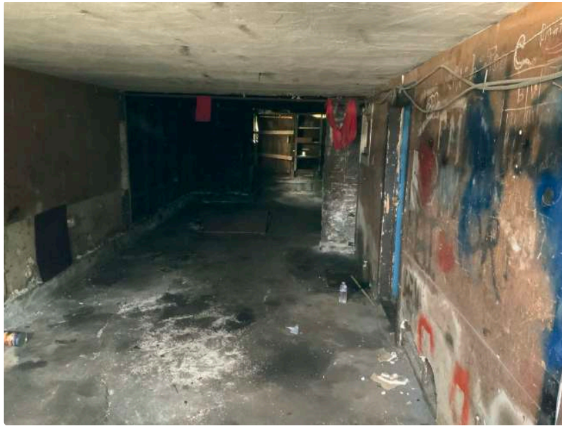
Interior of Subject Property; Garage; Facing East
