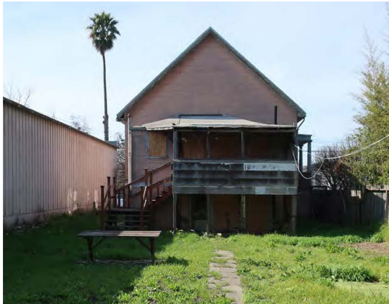
Fig.4 – 2421 Fifth St., Rear (east)
