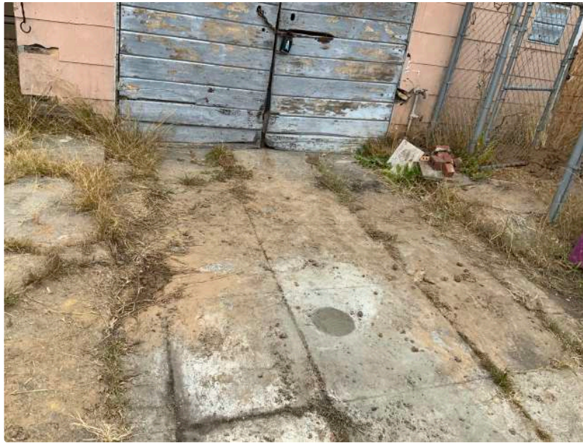
Exterior of Subject Property; Evidence of Geotechnical Boring
