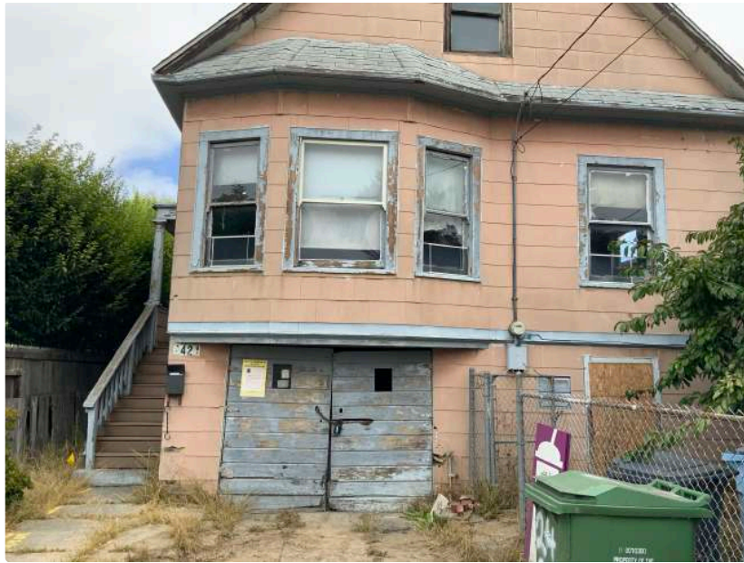
Exterior of Subject Property; Facing East
