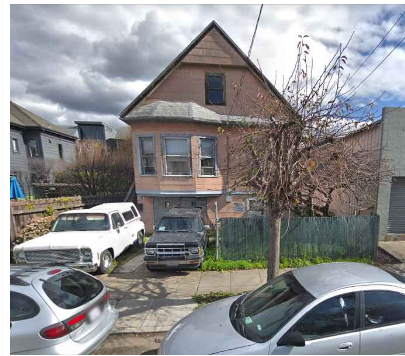
2421 FIFTH STREET, TO BE DEMOLISHED
