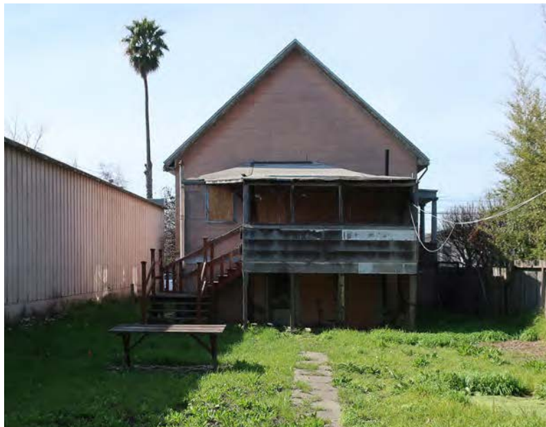
Fig.4 – 2421 Fifth St., Rear (east)
