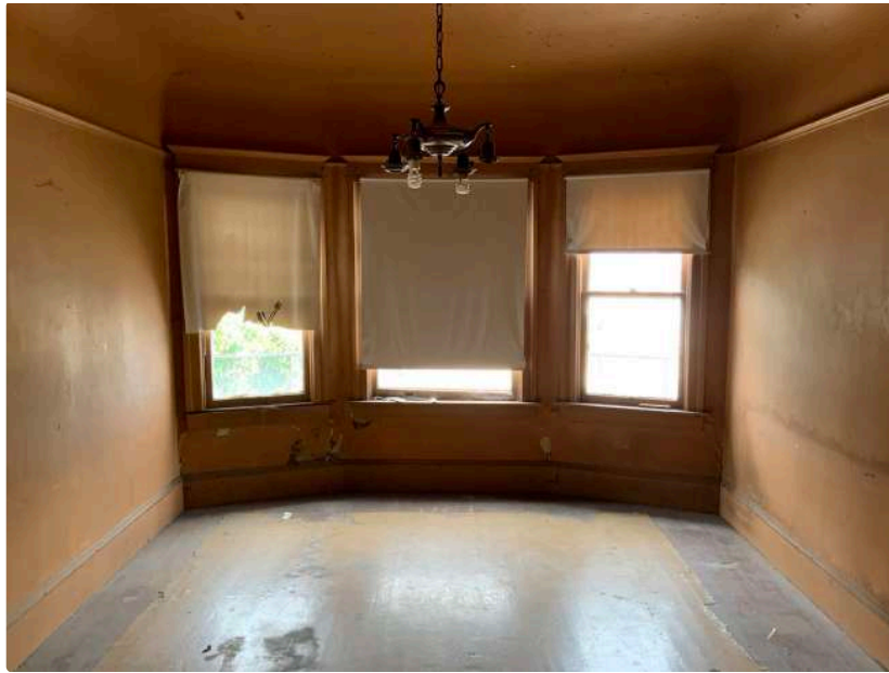
Interior of Subject Property; Facing West
