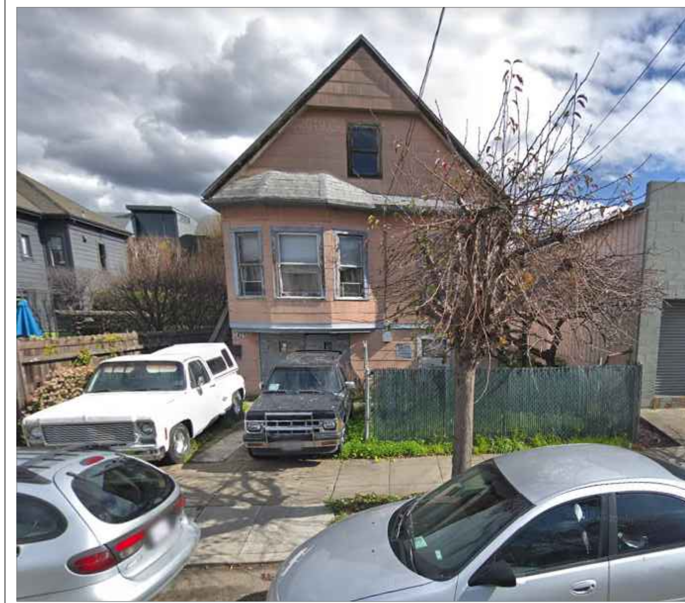
2421 FIFTH STREET, TO BE DEMOLISHED
