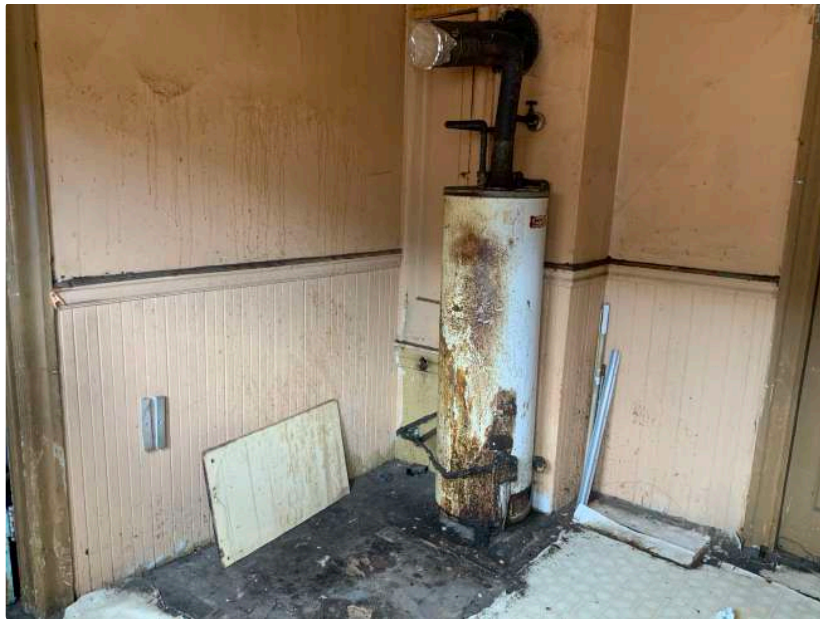
Interior of Subject Property; Facing North
